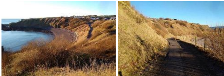
Figure 2. Left: Bay, slopes and cliffs affected by shallow landslides and surface erosion at OAL-UK; Right: Access road to the beach at OAL-UK.
